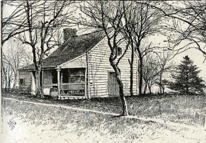
THE ROBINSON HOUSE. FROM A WAR-TIME PHOTOGRAPH.
